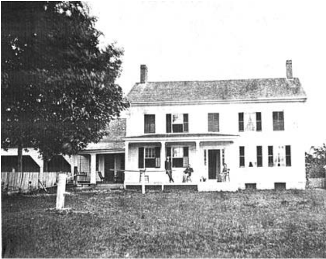
Original Dake home that burned on Daketown Road near Daketown School.
