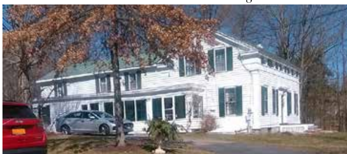
290 Locust Grove Road, April 2021
