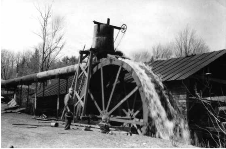
Kilmer's Water-Powered Sawmill, Middle Grove
