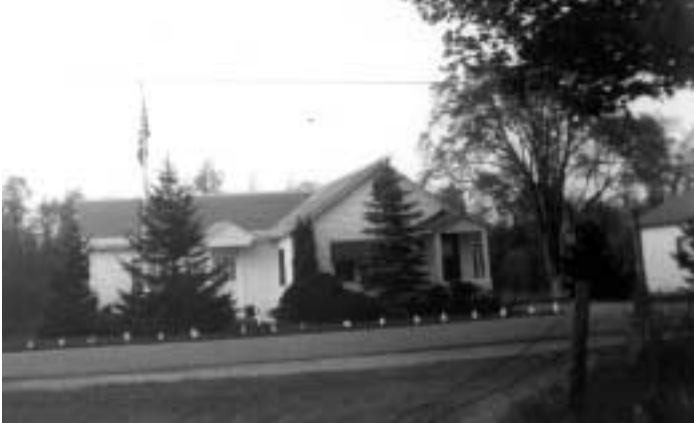
Post office after rooms built on so Ethel could live there.
