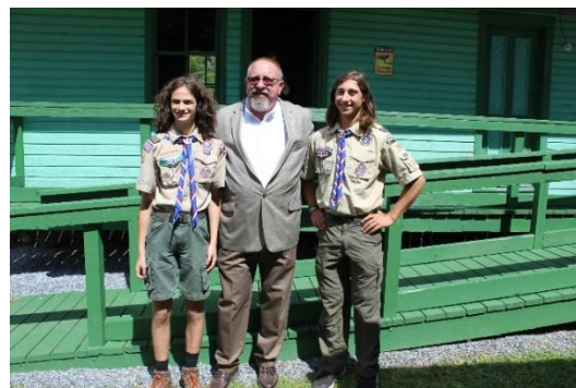
Seth Tremper, Kevin Veitch, Noah Szymanski Seth and Noah built ramps and stairs
