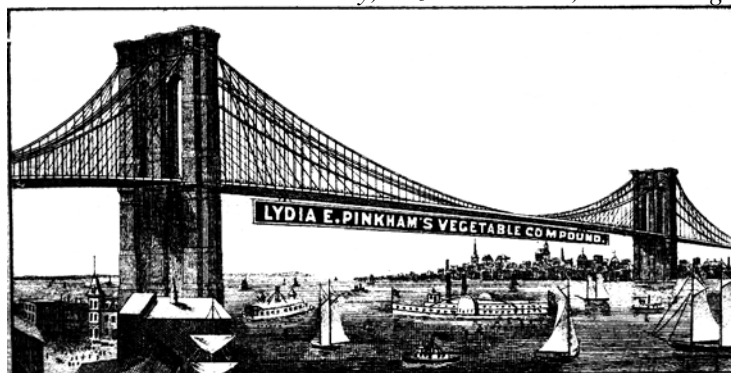
THE GREAT EAST RIVER SUSPENSION BRIDGE.
