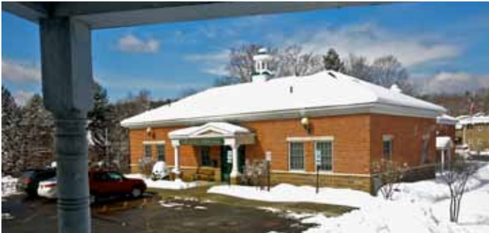
The Greenfield Town Hall 2013
